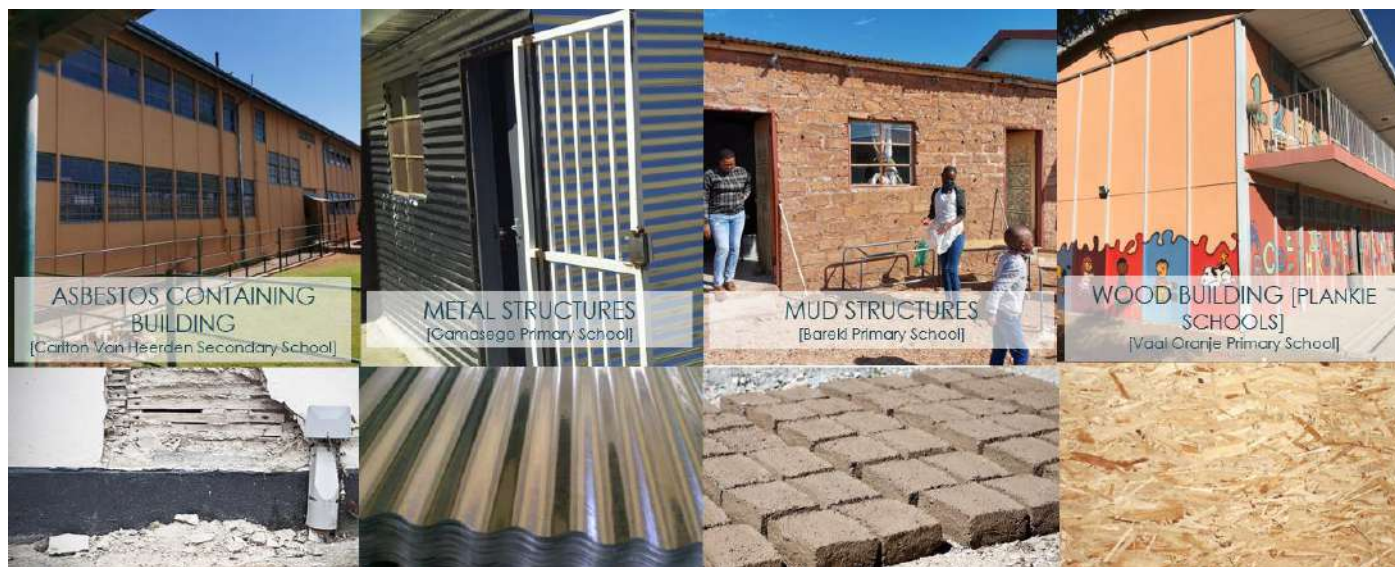
Figure 3: Inappropriate Structure Examples
